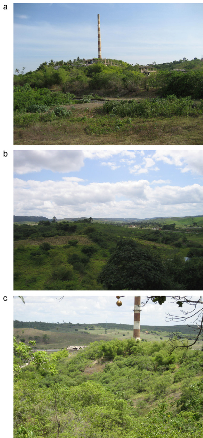
Fig. 2. (a) Lead smelter chimney stack and the concrete structure of the former plant, as seen from the road. (b) Slag heap showing the re-vegetating heap in the center and a pool that collects the rainwater (to the right of the concrete structure of the former plant). (c) The stack, the re-vegetating heap region, and the road.
